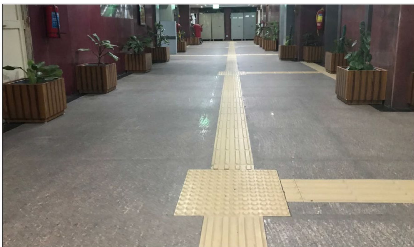
Example of Tactile Guiding Surface Indicators
