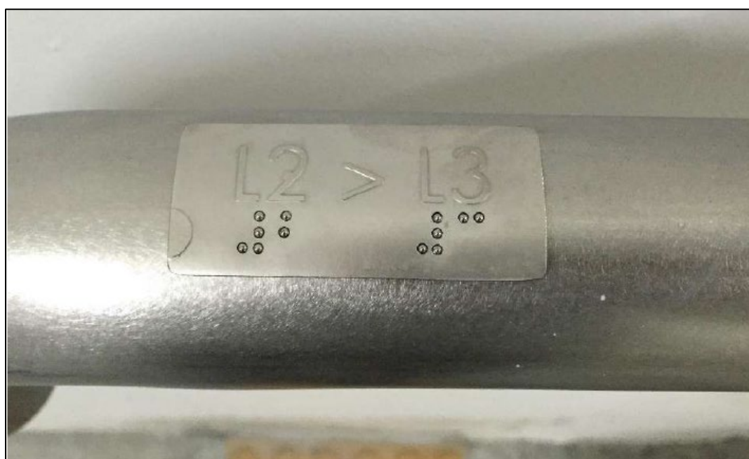
Braille indicators at end of the handrails
