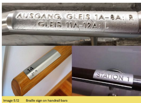
Image 5.12 Braille sign on handrail bars
