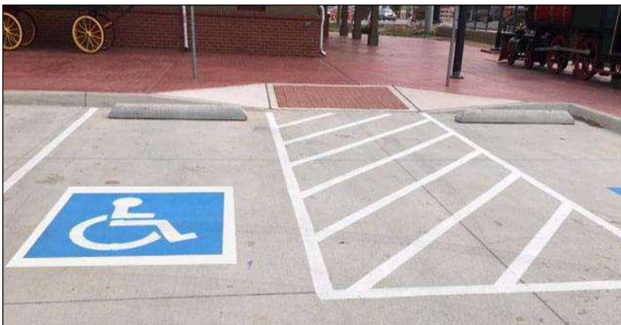
Example of parking symbol on floor, transfer bay marking and kerb ramp
