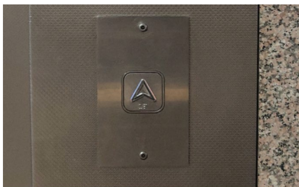
Image 5.4 Lift controls integrated with Braille Photo Credits: Dr. Gaurav Raheja
